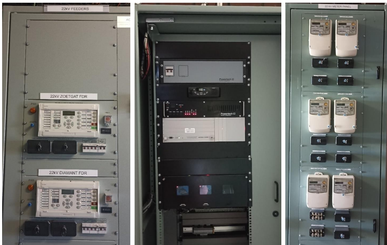
Figure 6: Disselfontein Rural substation's existing Protection, Telecontrol, and Metering equipment
